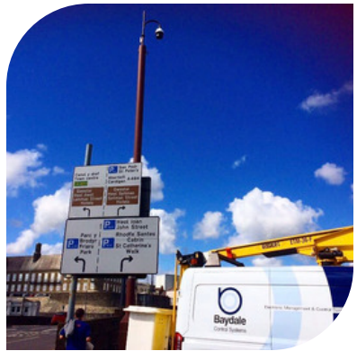
Baydale installing CCTV in Carmarthen
